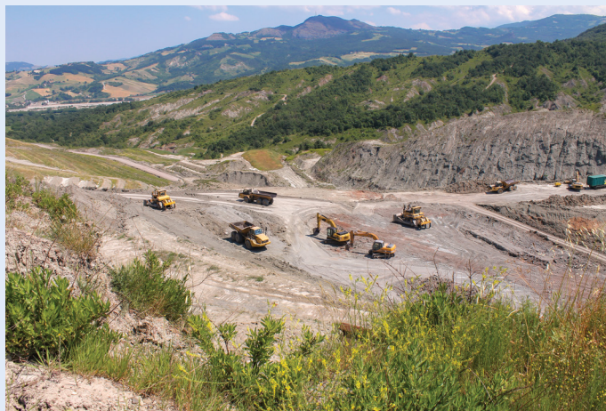
Figure 6: Construction vehicles changing the land.
